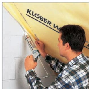
Wallint® 10 eco is a diffusible 2-layer air- and vapour barrier helping to improve the interior climate. Especially for timber boarded roof constructions or any boarded constructions without the use of counterbattens Wallint® 10 eco reveals its strengths. Due to its special coating Wallint® 10 eco prevents the ingress of humidity of the room into the insulation simultaneously offering a high degree of drying capacity and is CE-certified.
